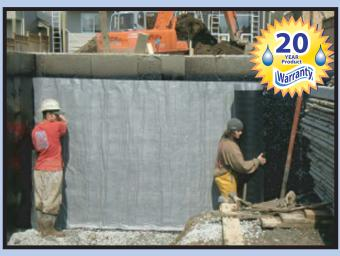
SUPERDRAIN Mats control water and drainage for above and below grade structures. Available in a variety of roll sizes produced for World Markets
